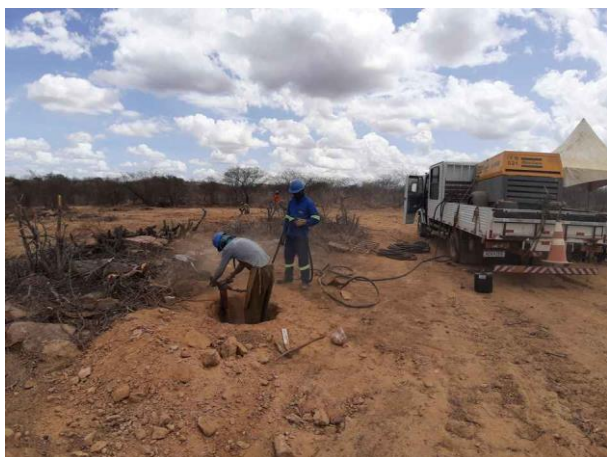
Figura 1. Torre 93/3, cava Central
