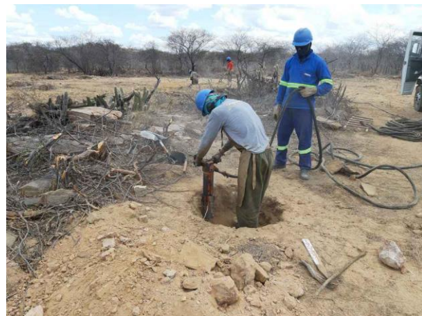
Figura 2. Torre 93/3, cava Central
