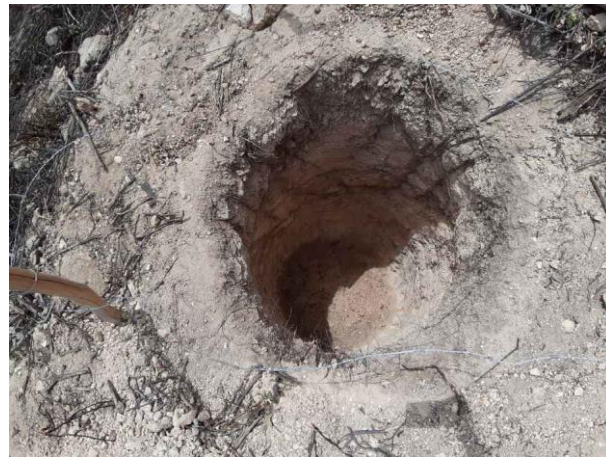
Figura 2. Torre 36/1, cava C.
